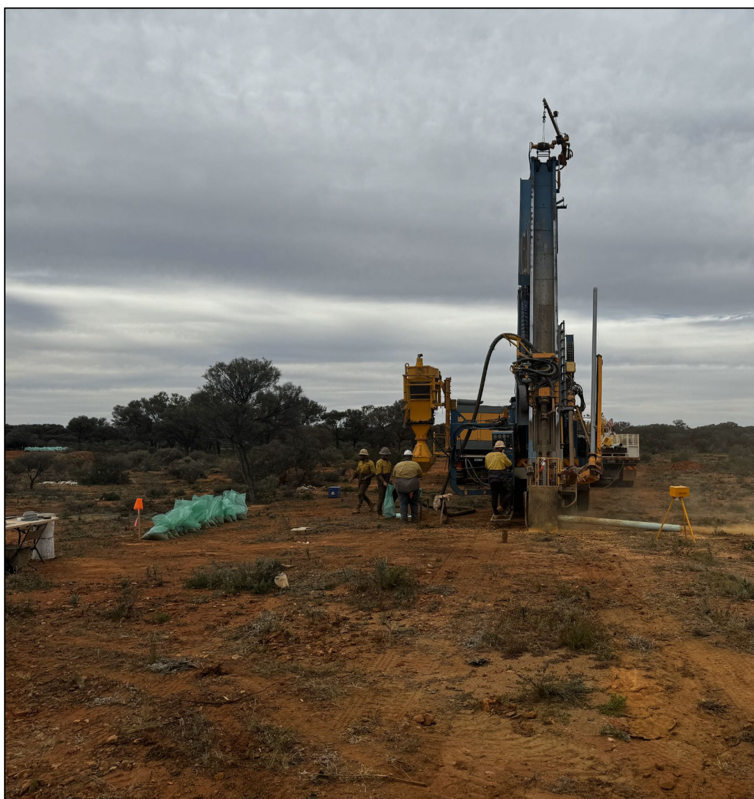
Figure 1. Challenge Drilling on site at Landed at Last, Yundamindra Gold Project.
